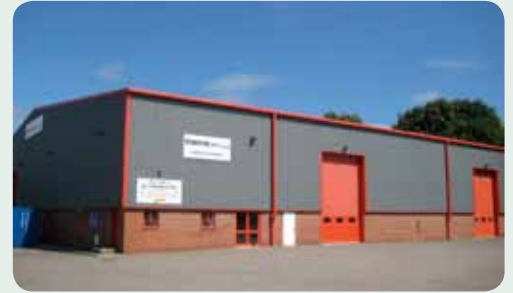
Transvac's new Research & Development Facility
