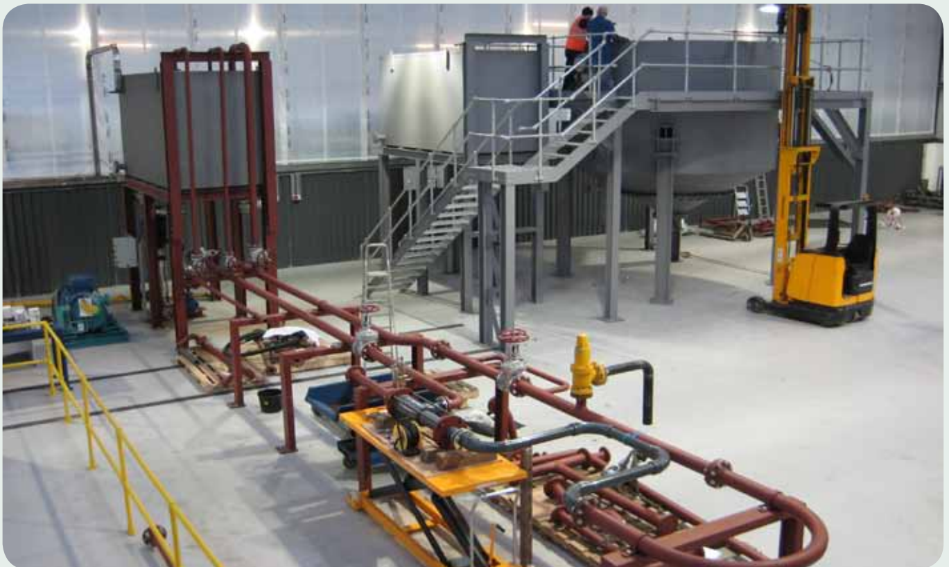
Transvac's new Research & Development Facility
